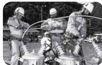
Page 24 THEN: Transformer exercise for the George Smith Shield 1987, Line Mechanics left to right: Doug Ashford, Henry Walker and Joe Clements
