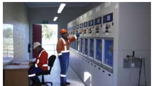
Te Rahu Substation from start to completion
