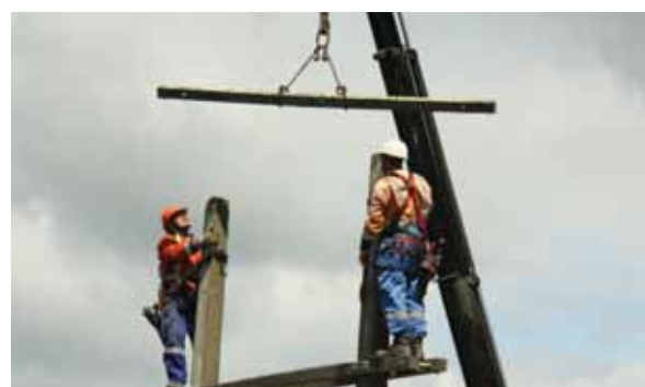
Horizon staff remove the poles after undergrounding of the power lines
