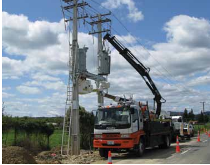
Hiab lifting one regulator into position
