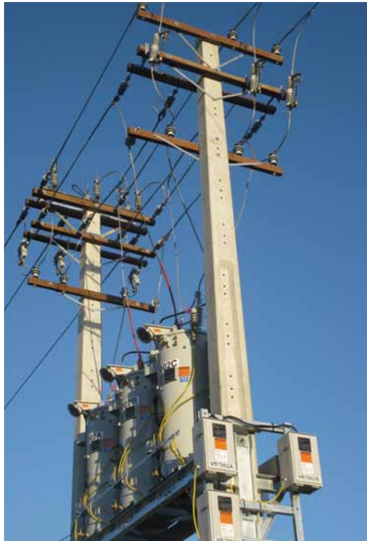
Completed three phase regulator and controllers
